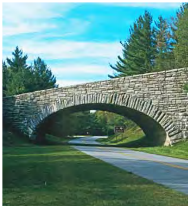
Bridges along the Blue Ridge Parkway are often constructed using native stones. The curved pattern of the key stones provides an added visual character. Image courtesy Library of Congress.
