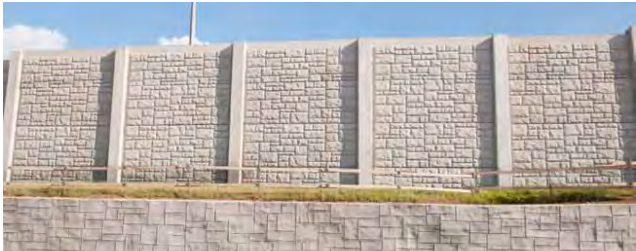
A noise wall is located at the top of a short concrete retaining wall that helps stabilize slopes and provides additional height to make the noise wall more effective. Image courtesy NCDOT.
