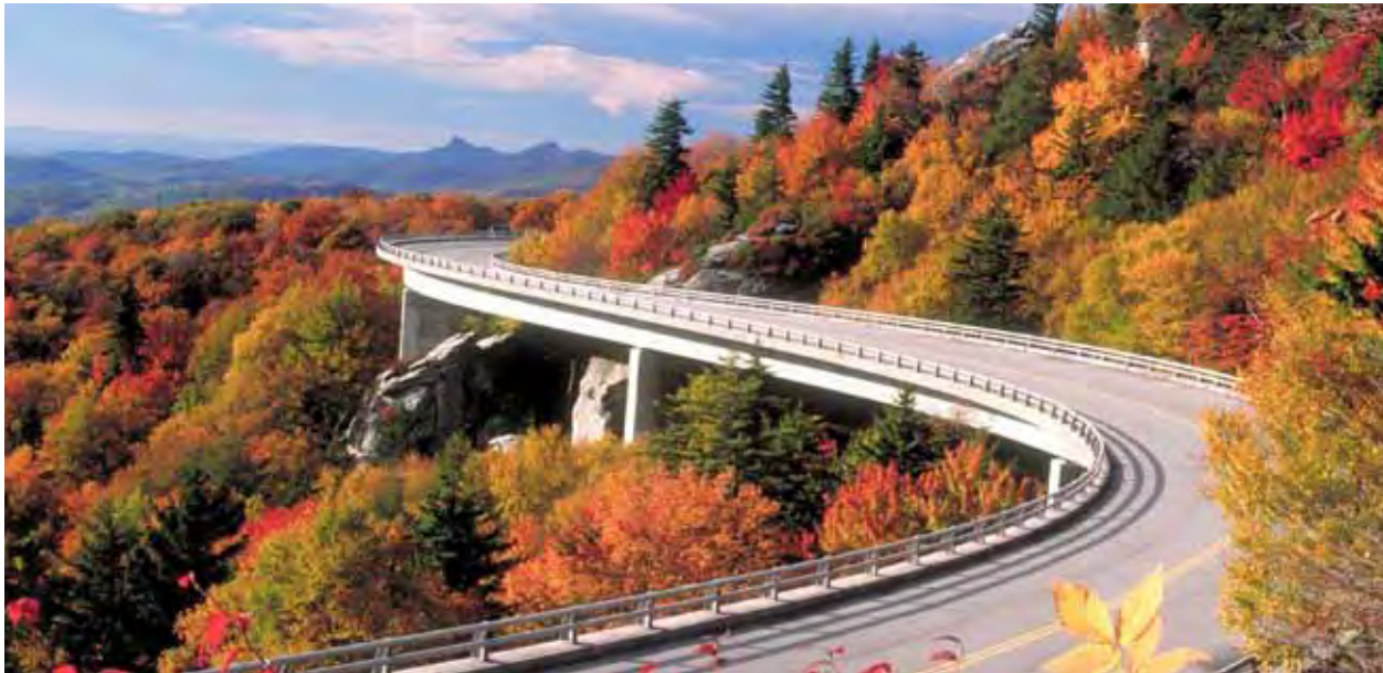
The Linn Cove Viaduct is one of the most photographed parts of the Blue Ridge Parkway. The viaduct is a 1,243-foot concrete segmental bridge that curves around Grandfather Mountain. It was completed in 1987 at a cost of $10 million and was the last section of the Blue Ridge Parkway to be finished. The Linn Cove Viaduct is recognized internationally as an engineering marvel. Image courtesy NPS public domain.
