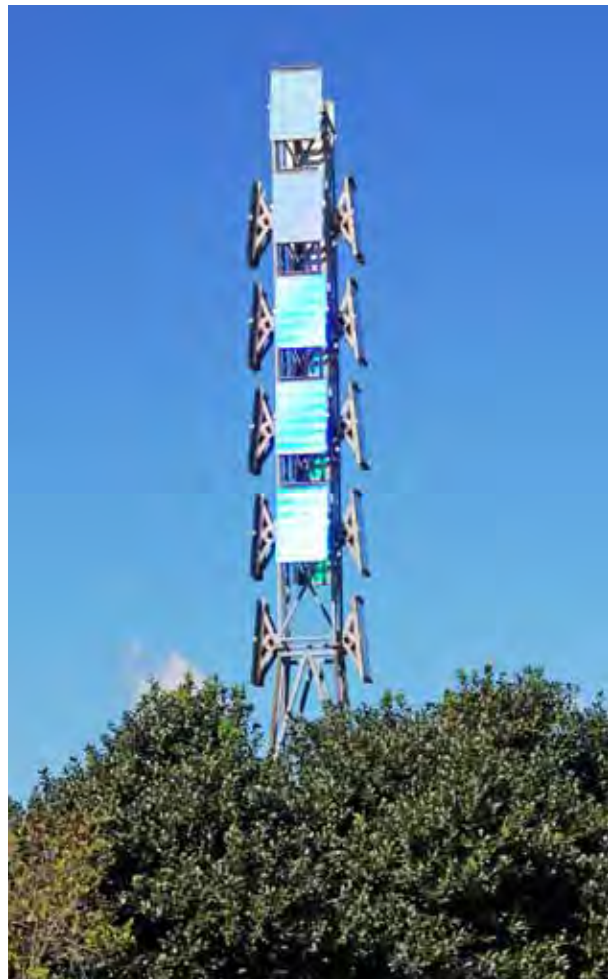
"Light and Time Tower" in Raleigh, North Carolina, was designed to diffract sunlight, visible to motorists driving along Capital Boulevard. Designed by Dale Eldred, this 40-foot tower is formed from 20 panels of clear glass. Image courtesy Mark Turner.
