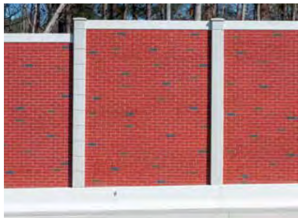
Brick noise wall along US 64, outside Apex, North Carolina. A brick pattern form liner was used to add visual interest. The grooves between and selected 'bricks' are painted to keep the wall from being too monotone in color and texture. Image courtesy NCDOT.
