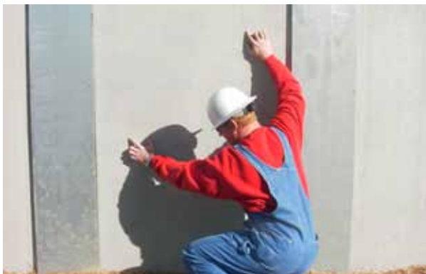
Precast concrete panel with galvanized steel H-piles. Image courtesy NCDOT.
