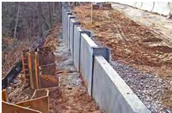
A retaining wall constructed of metal piers and precast concrete walls helps create a stable base for a new road. Image courtesy FHWA.
