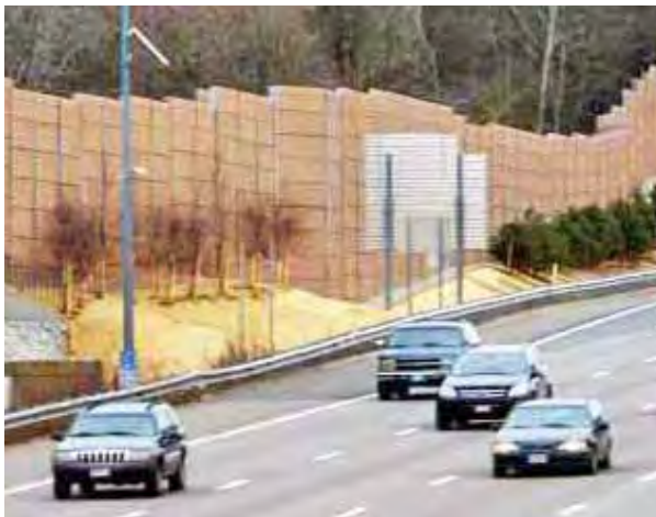
The jagged, uneven top of this noise wall is visually distracting and overly complex. Image courtesy FHWA.
