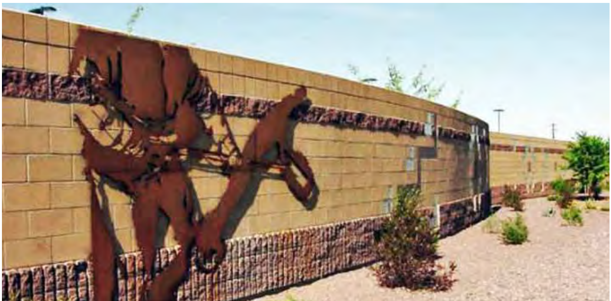
In the City of Glendale, Arizona, metal wall art is fastened to noise walls. The walls are made of tan-colored concrete masonry units, with a stone veneer used at the base and near the top of the walls. Image courtesy Creative Design Resolutions.
