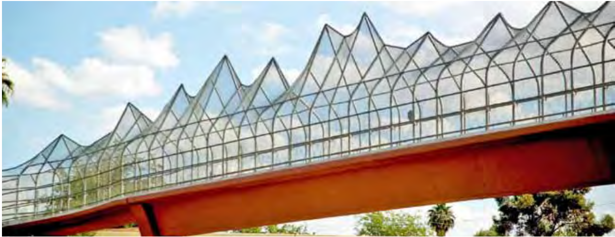
The Mountain Pass along Highway 51 in Phoenix, Arizona, was inspired by the jagged profile of the nearby Piestewa Peak Range. Vines climbing on the chain link fencing transform the safety cage to shade element. Artist Laurie Lundquist designed in collaboration with SVR Inc. Structural Engineers and HDR Inc. Image courtesy Laurie Lundquist.
