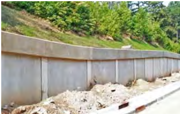
Precast concrete panel with steel H-piles facing. Piles painted gray, not a standard NCDOT practice. Image courtesy NCDOT.
