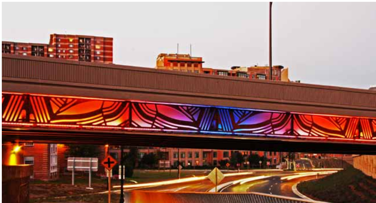
Design motifs used for the Arlington, Virginia Boulevard bridge were inspired by native redbud trees. Heart-shaped leaf patterns and seed pods add texture, and laser-cut leaves are LED back illuminated with programmable reflecting sky tones. The project was designed by Vicki Scuri SiteWorks with AECOM Transportation. Image courtesy Vicki Scuri.
