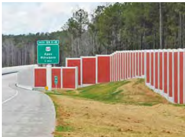
Brick noise wall along US 64, outside Apex, North Carolina. A brick pattern form liner was used to add visual interest. The grooves between and selected 'bricks' are painted to keep the wall from being too monotone in color and texture. Image courtesy NCDOT.
