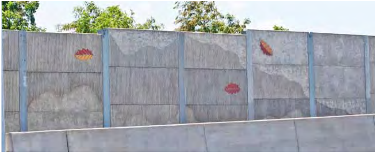
The fluted patterns on these precast concrete panels represent the surrounding mountains in Asheville, North Carolina. This technique and level of integration can be considered a landmark noise wall type. Image courtesy NCDOT.
