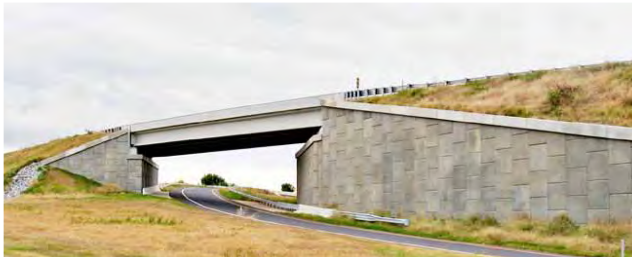
These precast panels are used to create an abutment for this bridge. Image courtesy FHWA.
