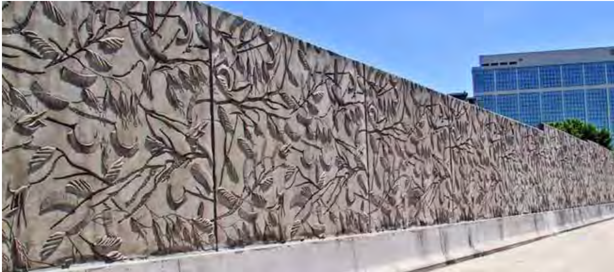
Precast concrete panels - Surface treatment of retaining walls and noise walls for Denver's Transportation Expansion Project of the I-25 Corridor were designed by artist Carolyn Braaksma using precast concrete panels. The artist developed patterns and images for precast concrete retaining and noise abatement walls. Image courtesy Carolyn Braaksma.
