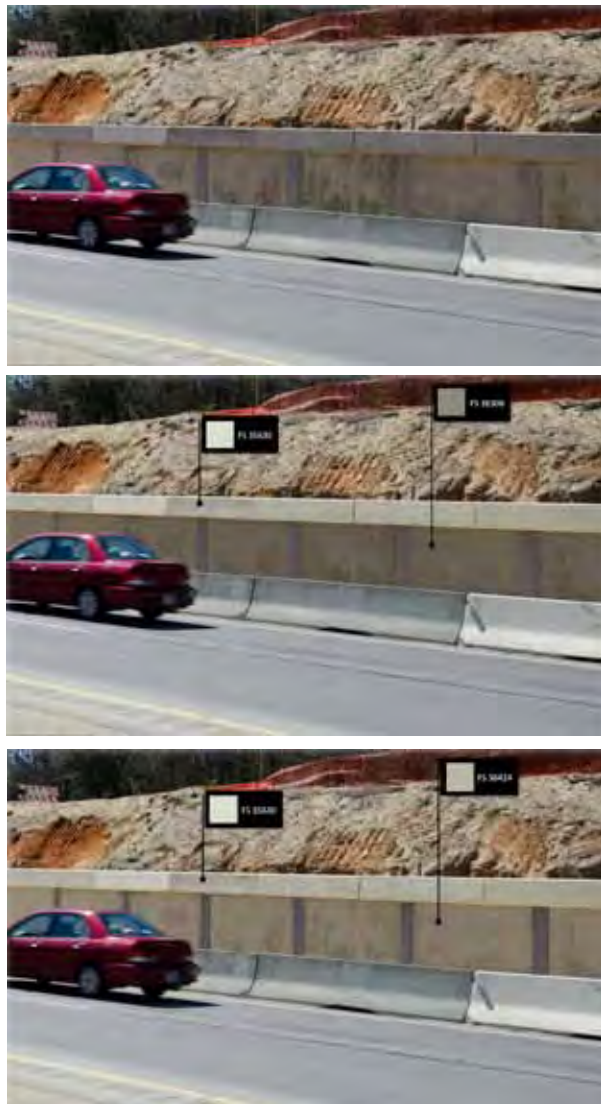
This sequence shows an existing retaining wall (top) and two visual simulations (bottom images) showing the use of concrete stains. Images courtesy NCDOT.
