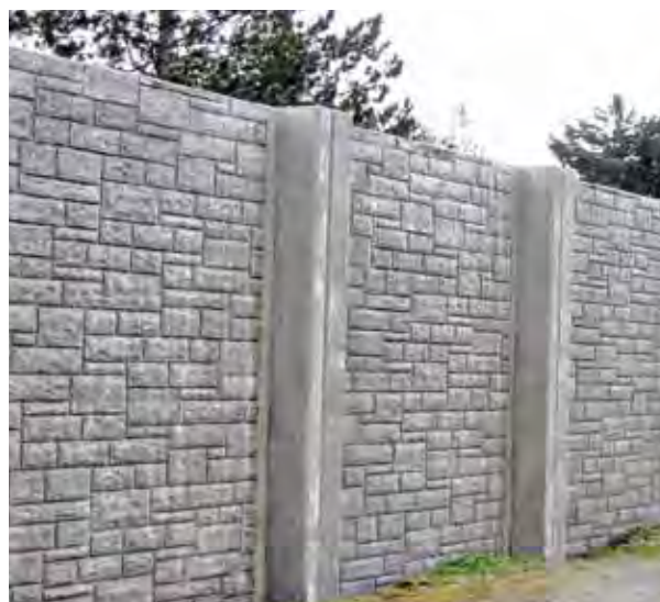
This concrete wall uses form liners to create an Ashlar Stone pattern, and both the panels and concrete piers are stained to create a more muted color. Image courtesy FHWA.
