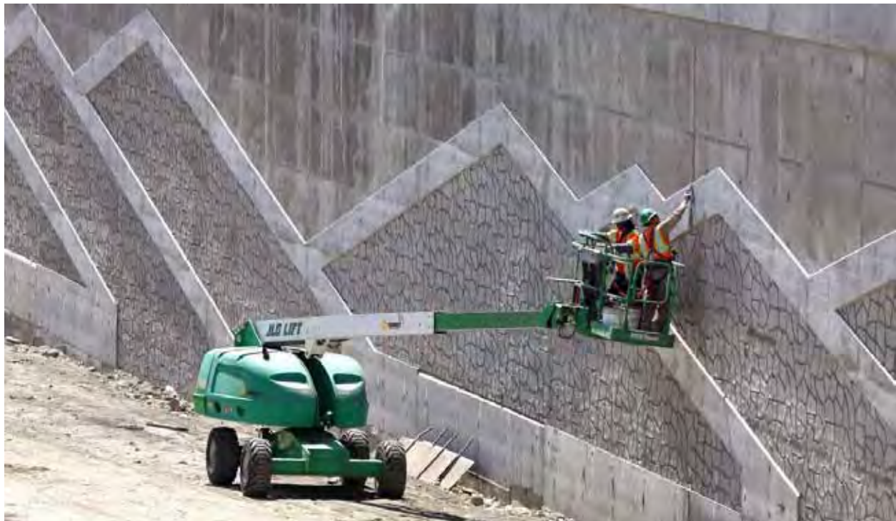
Construction of a noise wall along I-5 in Santa Clarita Valley, California. Triangular patterns reflect the surrounding mountains. Image courtesy California Department of Transportation.
