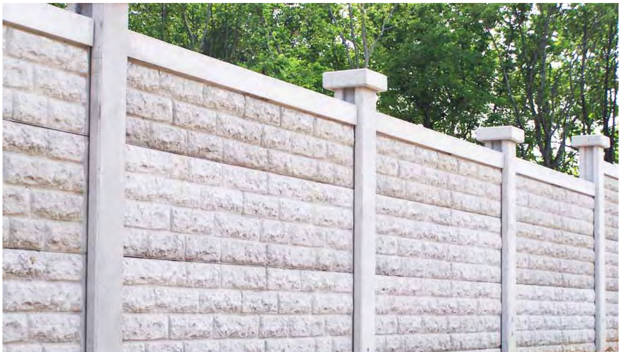
Concrete piers support precast concrete panels with stone patterns created with form liners. The cap gives the wall a finished appearance. Image courtesy NCDOT.
